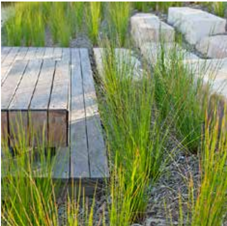
Timber deck in rain gardens
